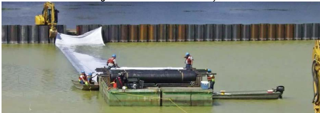
Figure 3-3. Placement of a Clay Mat
