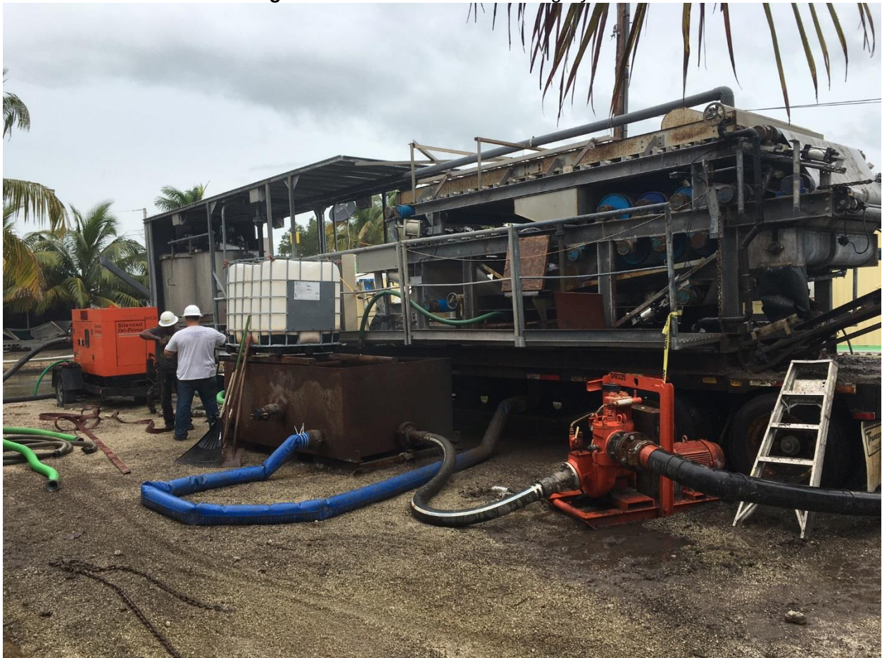
Figure 1-2. Mechanical Dewatering System
