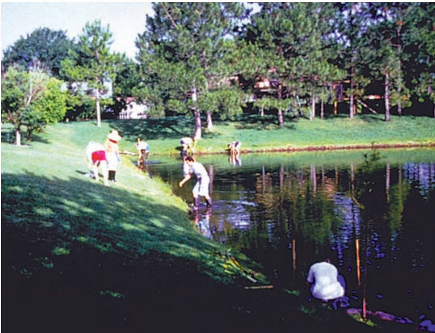
Residents aquascaping their wet detention pond.
