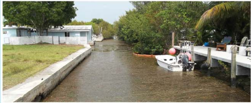
"Poor" water quality conditions have been noted in the canal between Witters and Baileys Lanes in Doctors Arm in Big Pine Key.
